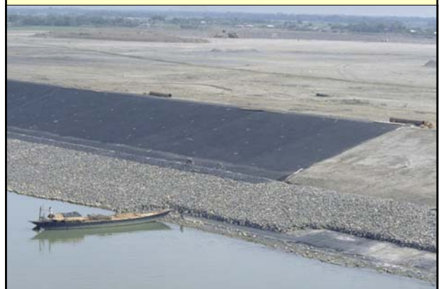
RIVER BANK PROTECTION
