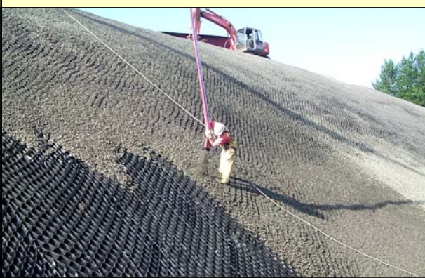
GEOCELL ON STEEP SLOPE
