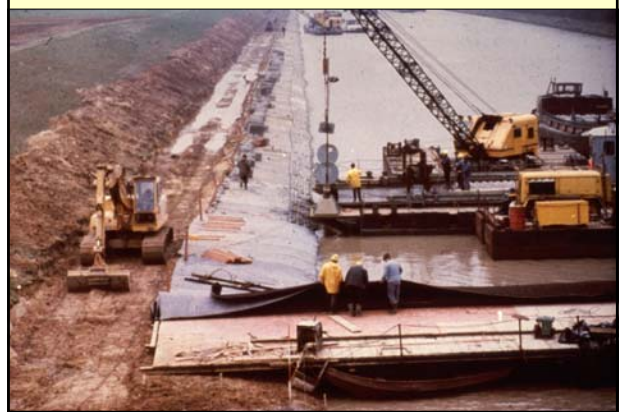
CANAL BANK PROTECTION
