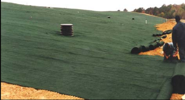
Geomat rolls used for erosion control
